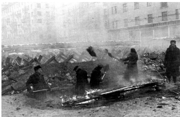
The erection of fortifications on the streets of the capital
