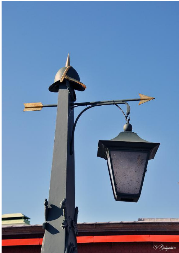
Lamps and fragments of a decor of a protective lattice of Ioannovsky Bridge
